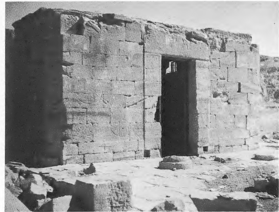
Plate 34. Façade of the temple of Nekhebet at El Kab.
